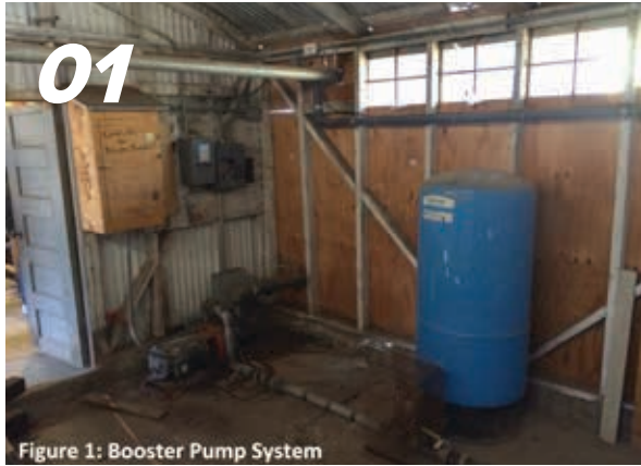
Figure 1: Booster Pump System
