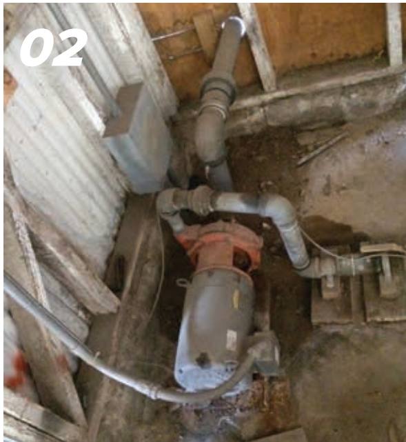
Figure 1: Booster Pump System
